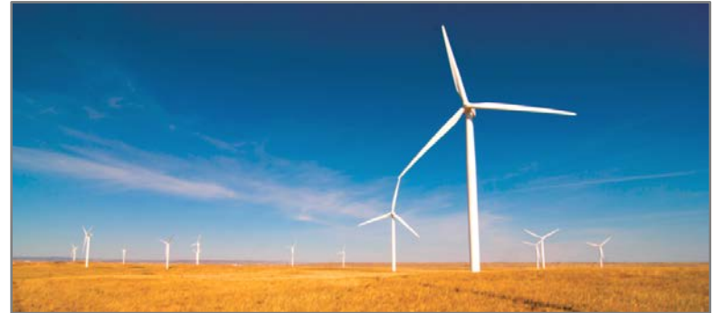
Pictured: Happy Jack Wind Farm located near Cheyenne, Wyoming, serves Wyoming and South Dakota Electric (owned by Duke Energy)
