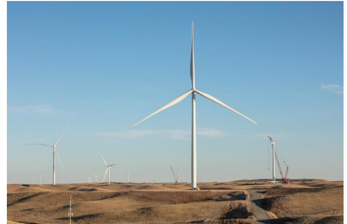
52.5-Megawatt Corriedale Wind Energy Project near Cheyenne, Wyoming
