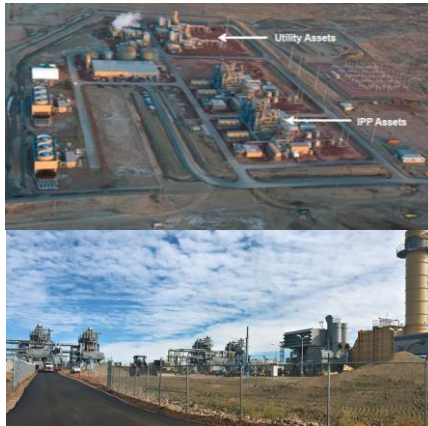
Pueblo Airport Generating Station
