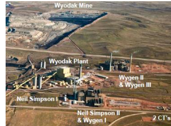
Gillette Energy Complex
