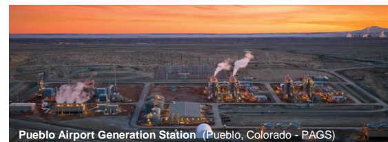
Pueblo Airport Generation Station (Pueblo, Colorado - PAGS)
