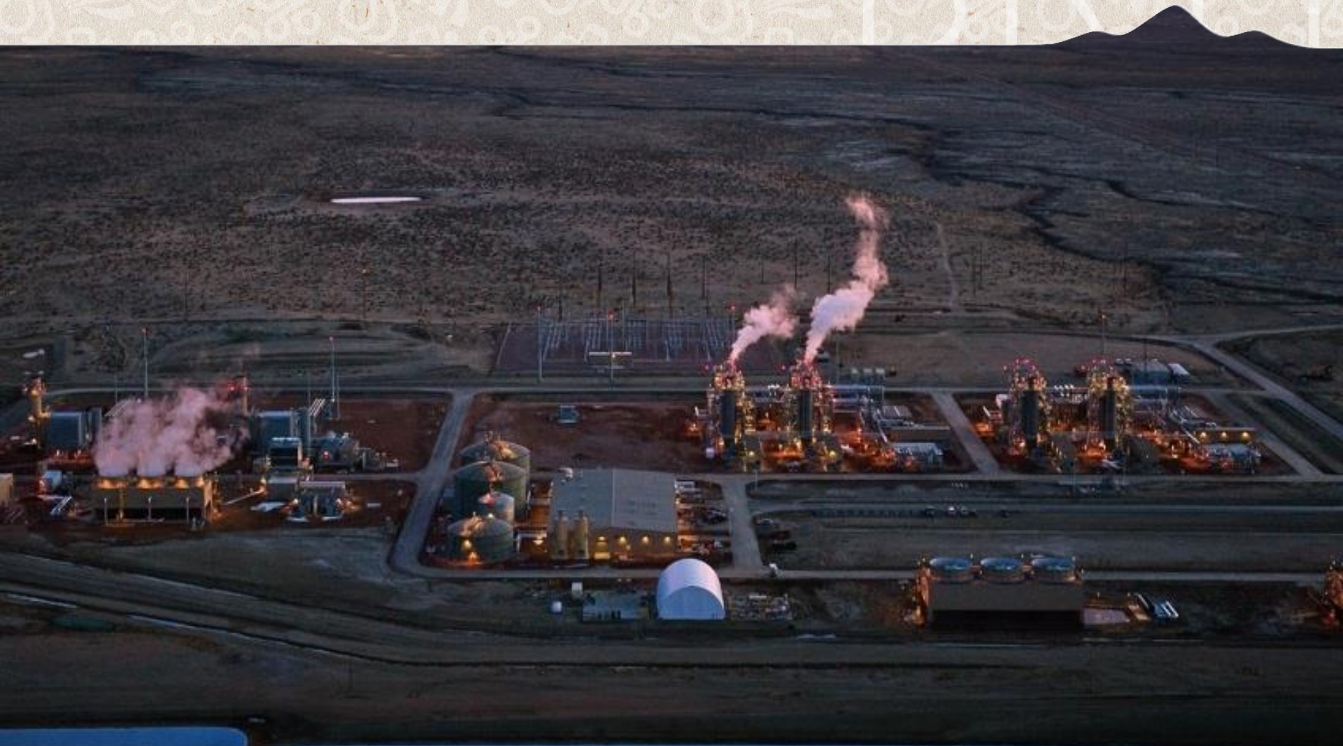
Pueblo Airport Generating Station near Pueblo, Colorado
