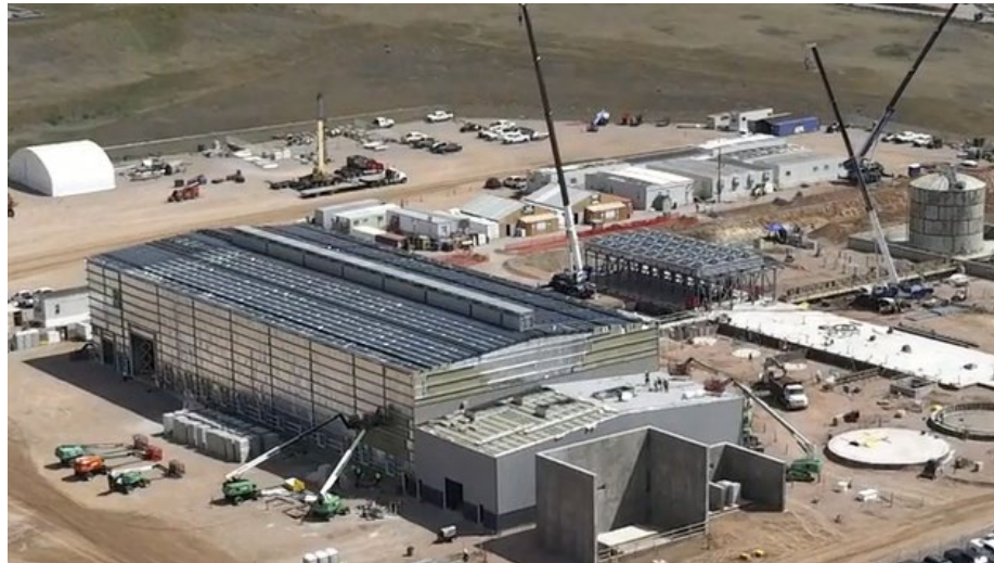
Pictured: Lange II generation project site under construction in Rapid City, South Dakota
