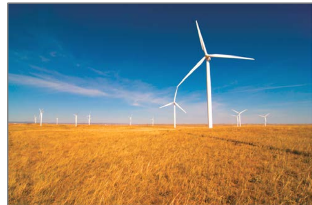
Pictured: Happy Jack Wind Farm located near Cheyenne, Wyoming, serves Wyoming and South Dakota Electric (owned by Duke Energy)
