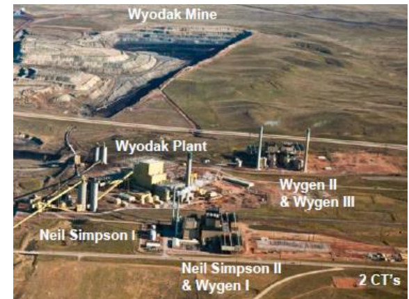
Gillette Energy Complex
