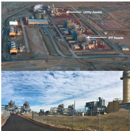
Pueblo Airport Generating Station
