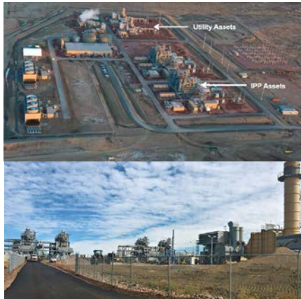
Pueblo Airport Generating Station
