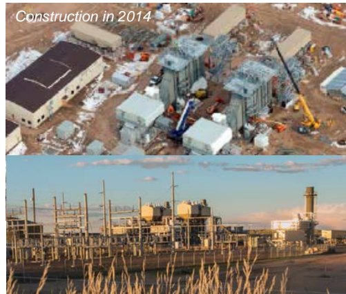
Cheyenne Prairie Generating Station
