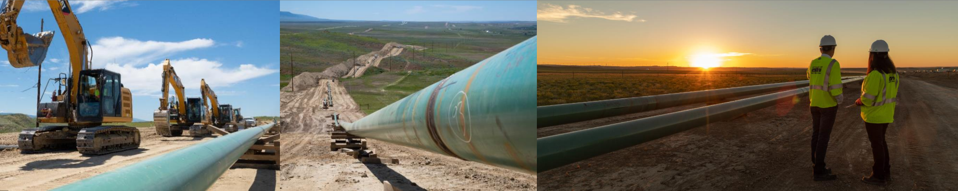
35-mile Natural Bridge pipeline - Central Wyoming
